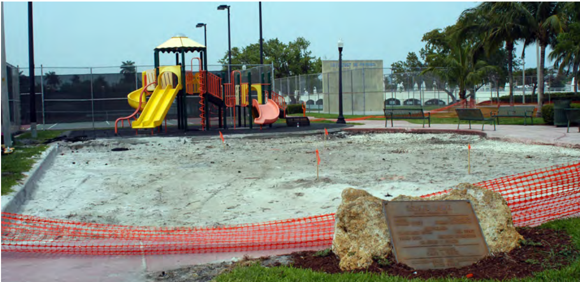
Palm Island Park: under construction - May 2007
